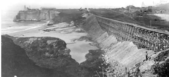
Ocean Shore rail trestle south of Davenport. The wooden structure still exists under loads of dirt fill that was dumped alongside to stabilize the trestle.
